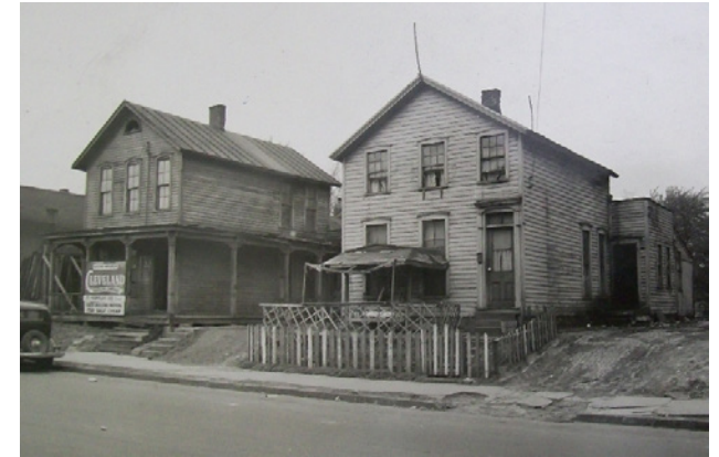
1930s view of early homes along Nebraska Avenue. These were among the most ubiquitous house types of the 1860s and 1870s. The home at the right had modest Greek Revival influence, namely in the corner entrance with pilasters and pedimented window hoods. The house on the left contains elements of the Folk Victorian style, namely the L-shaped porch with decorative columns and mouldings.
