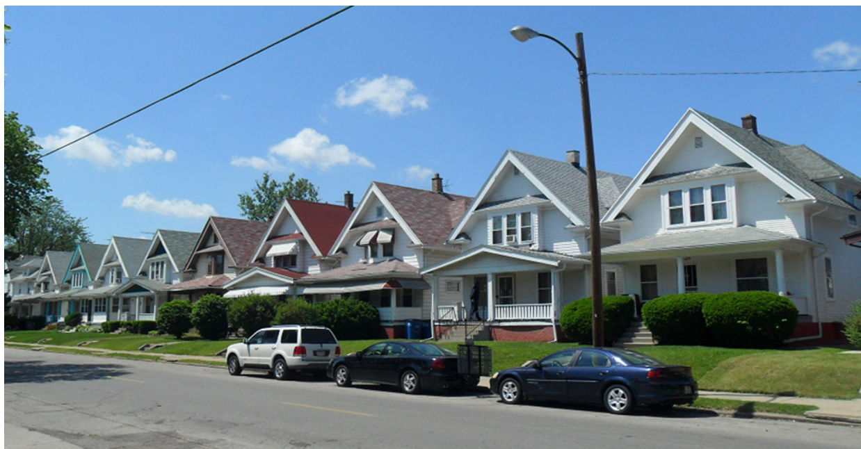
1000 Block of Indiana. Built in the mid 1920s, these houses are a part of a three-block plat extending to Dorr Street which was one of the last significant development of single family homes until the urban renewal era of the 1960s.
