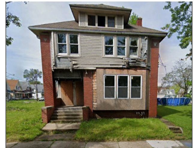
Dilapidated Housing in Junction
