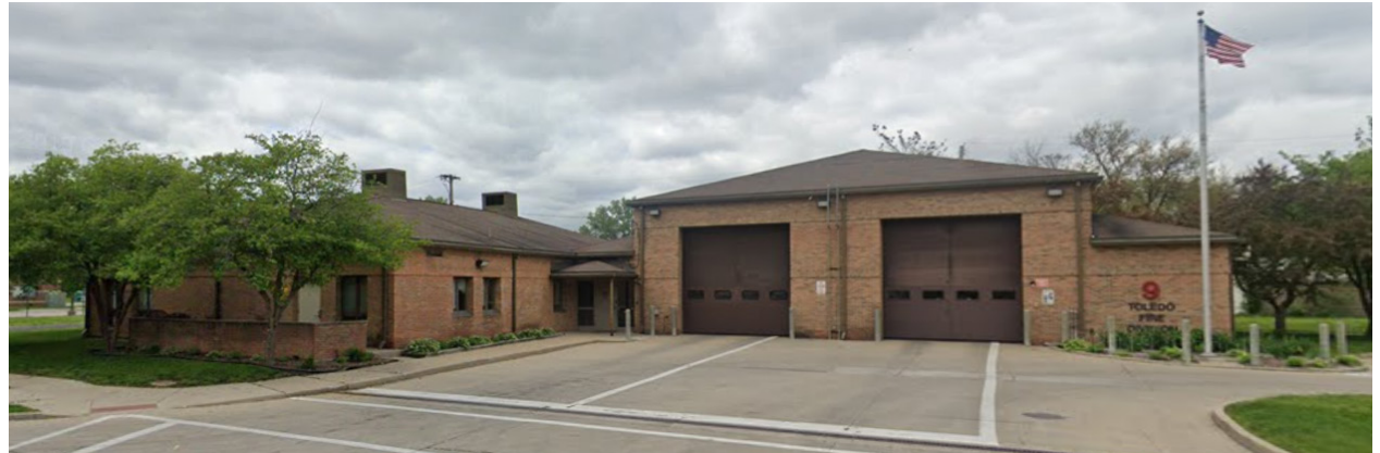
Existing Fire Station.
