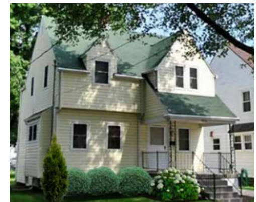
LHSC Rehabbed Housing
