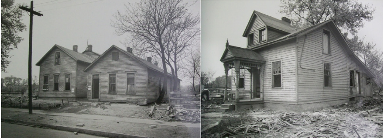
The few remaining old wood-framed houses awaiting demolition for the Brand Whitlock Homes, late 1936
