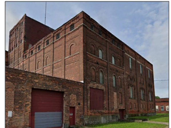
Existing industrial building for adaptive reuse.
